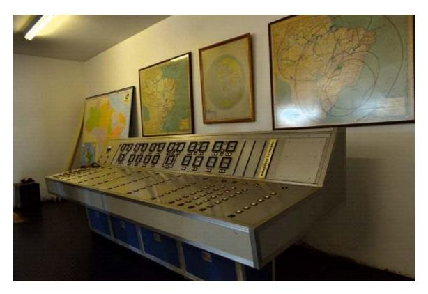
By this console (above) we can see different maps with the radiating lobes of the antennas, and the theoretical coverage of transmissions from different areas of Brazil and the world.
